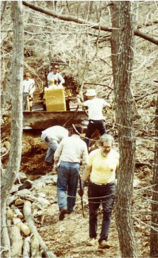
Winter 1979 - Harold Crate and others create part of the access road to the cabin site - someone brought their bulldozer
