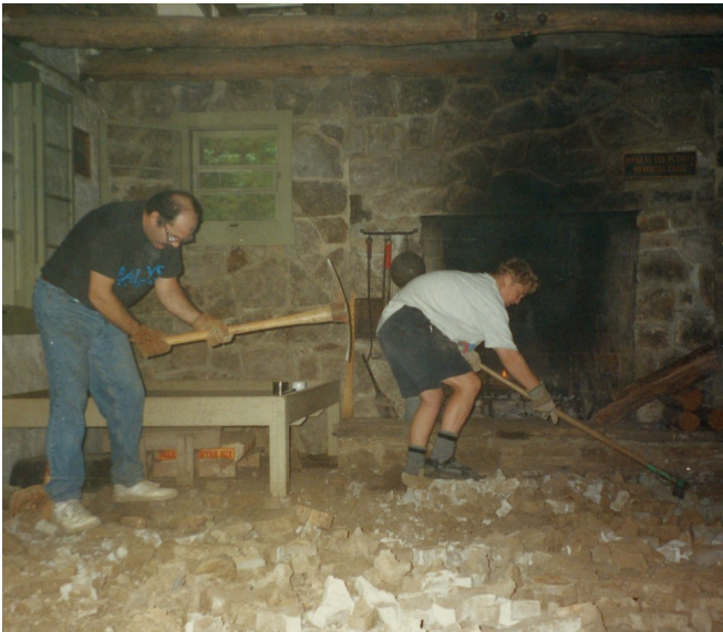
September 1995 - Steve Babor and Dan Barham breakup and remove the original cabin floor
