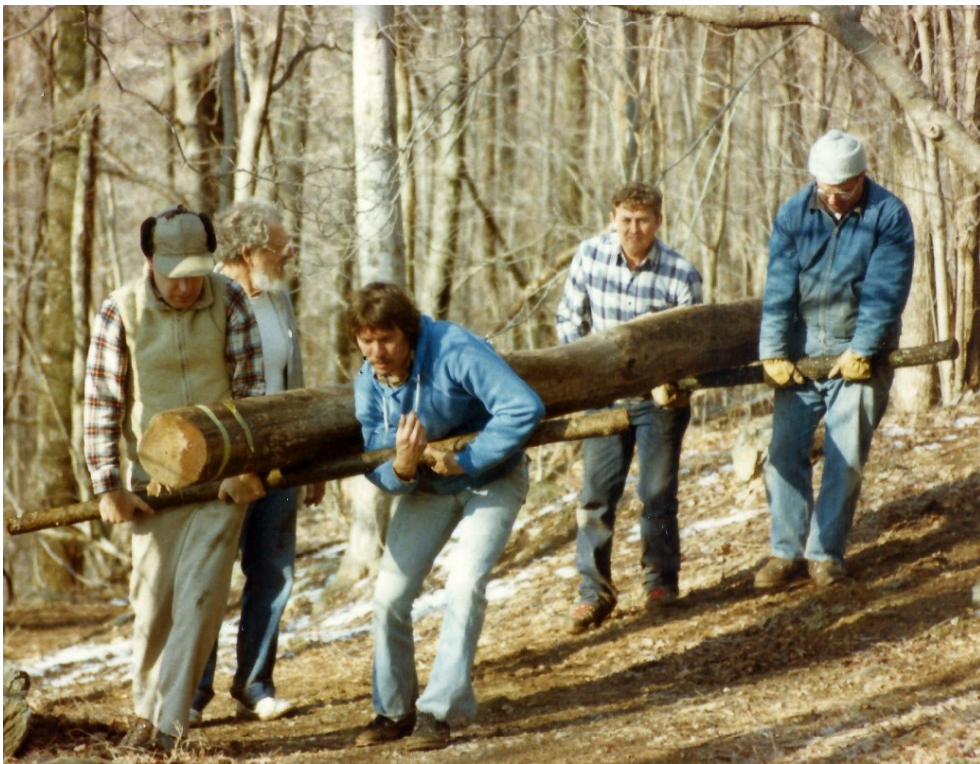
March 1985 - Carrying a log for the underpinning of the front porch - Mark Connolly, Harold Crate, Bob Adkisson, Jerry Burch, and Bill Newsom
