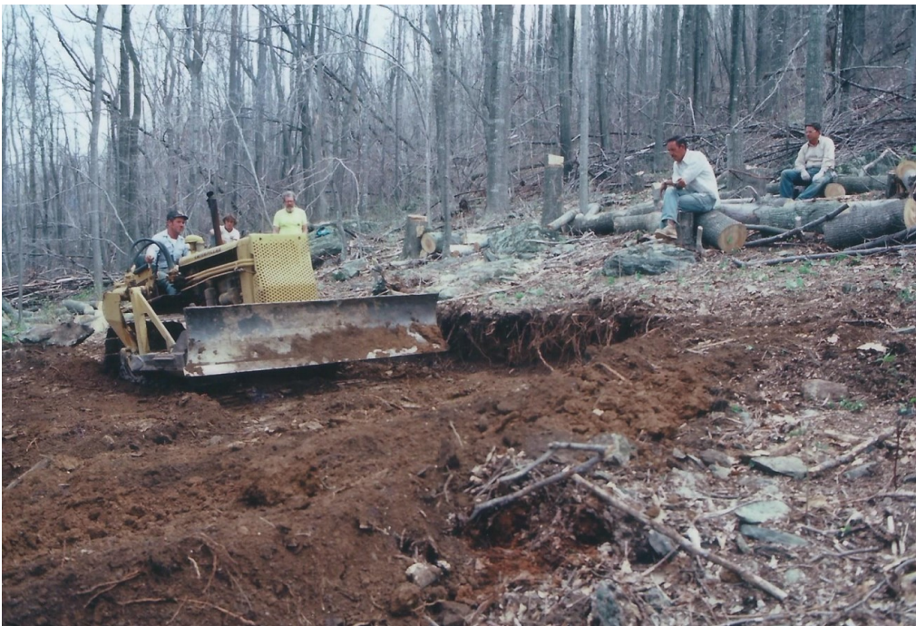
Bulldozing Cabin Site Clearing
