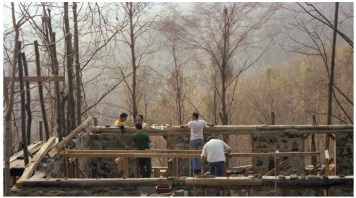
Cabin Walls going up 1981
