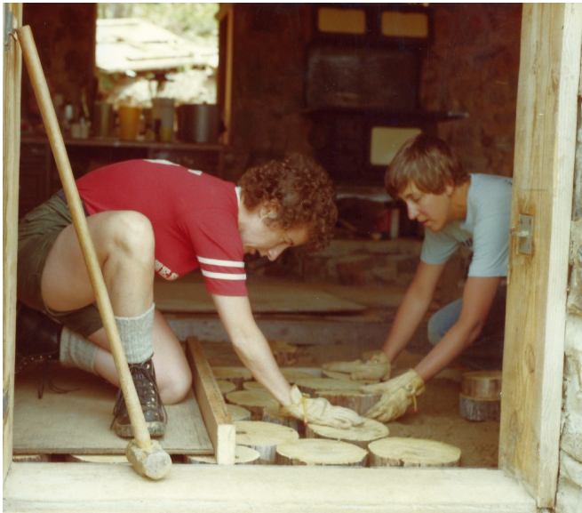
May 1983 - Linda Campbell and Nancy Barger lay tree rounds in mortar - the original cabin floor
