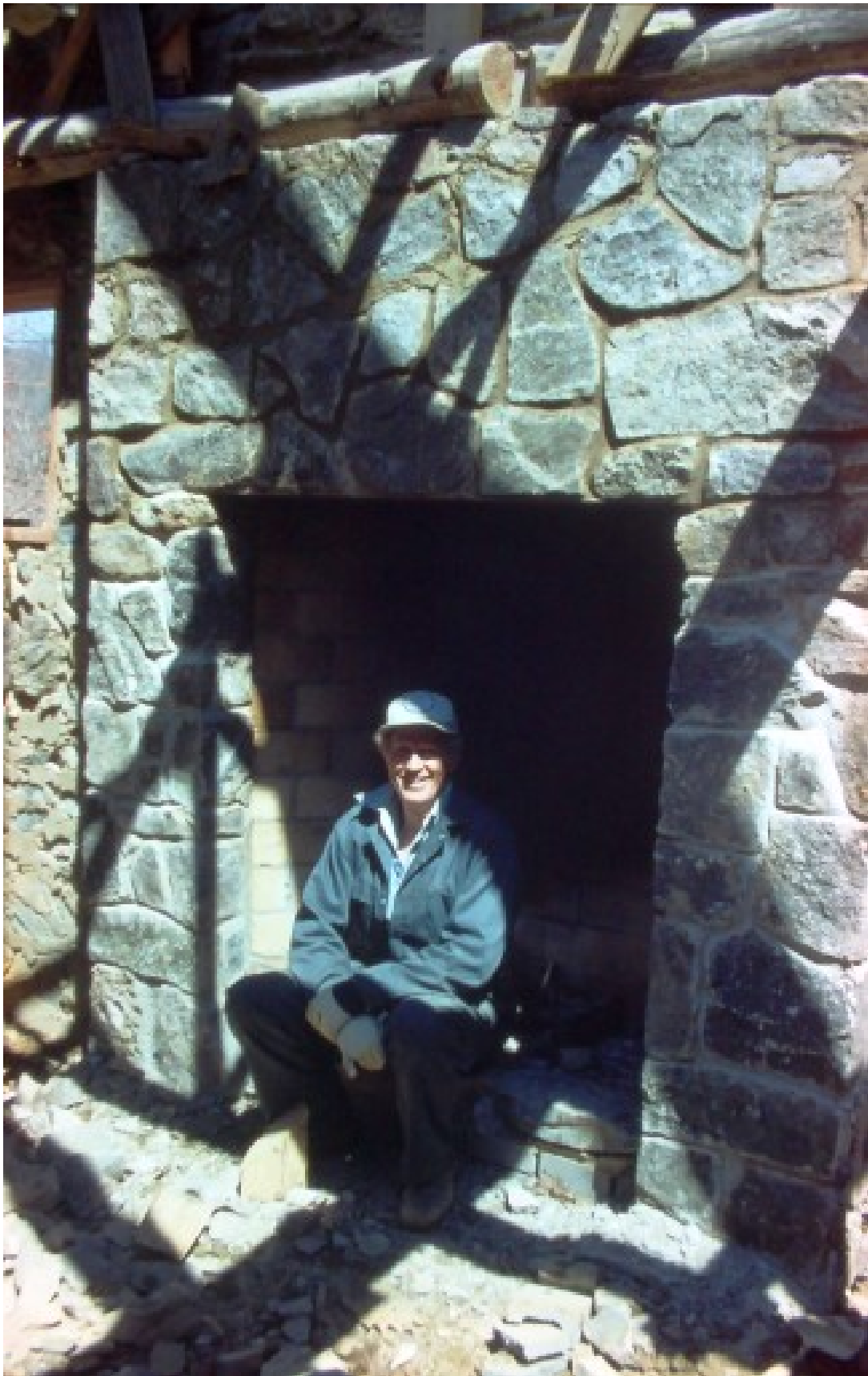
April 1982 - Otey Shelton supervised the laying of stones - He did the work on the fireplace himself
