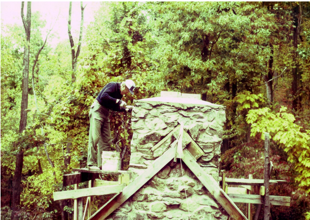
October 1981 - Otey finishes the Big Chimney
