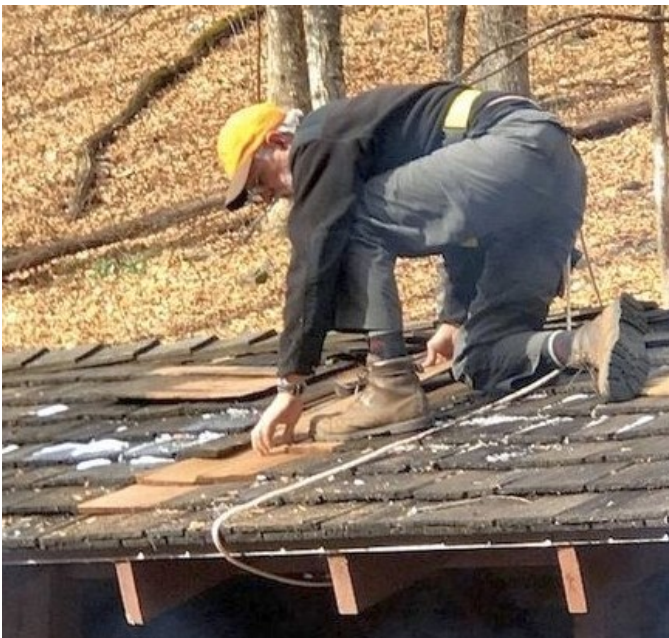
Milton Beale repairing Harpers Creek Shelter Roof
