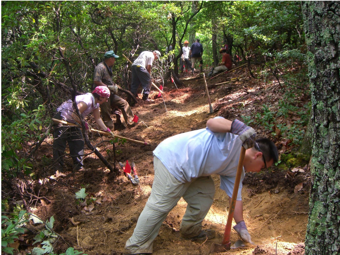
TATC Members & Konnarock Crew relocating section of TATC's Trail
