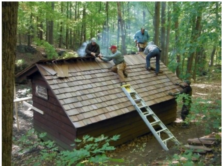
Harpers Creek Shelter gets a new roof
