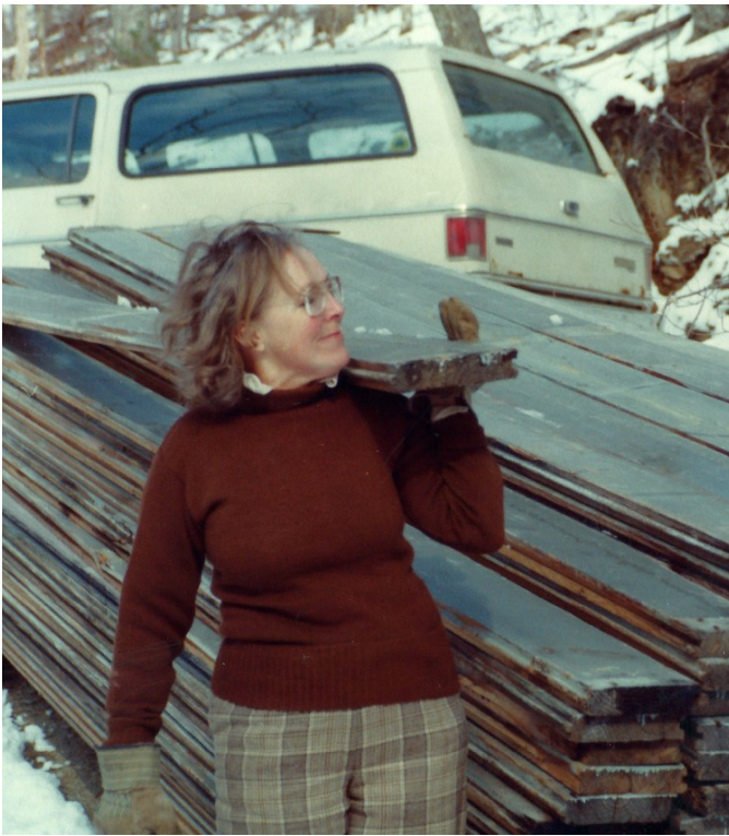
Winter 1982 - Marilyn Horvath about to carry a roof board to the cabin
