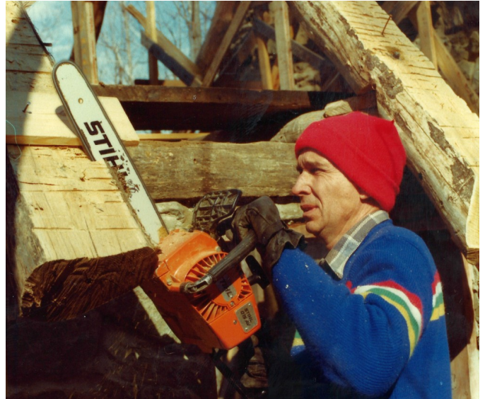
Early Spring 1982 - Karl Price trims the newly placed rafters
