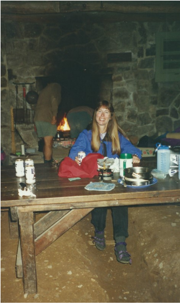
Jenny DeArmond at the TATC Cabin the weekend that a small crew removed the original floor
