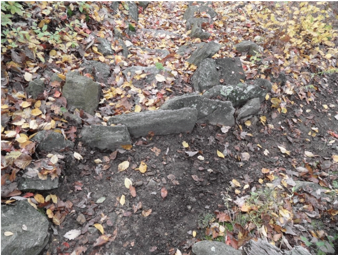
A Nicely Shingled Rock Waterbar after Maintenance.
