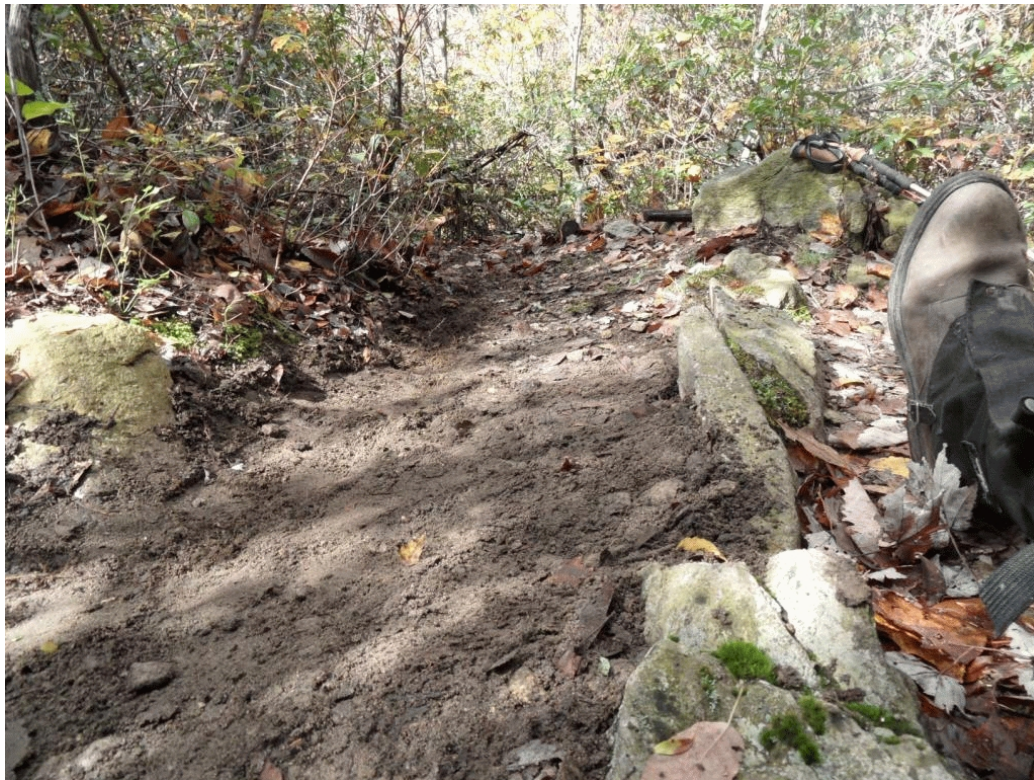
The Grand Prix Curve Diverts Water Away from the Waterbar into the Drainage Channel. Note the Slope of the Curve.
