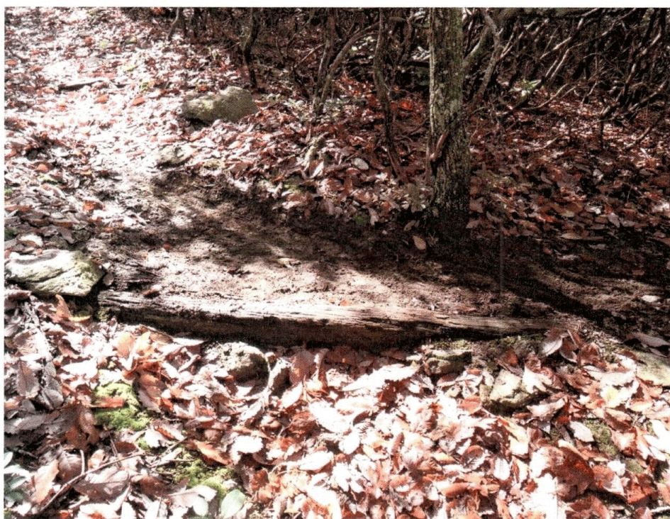
A Simple Waterbar after Maintenance
