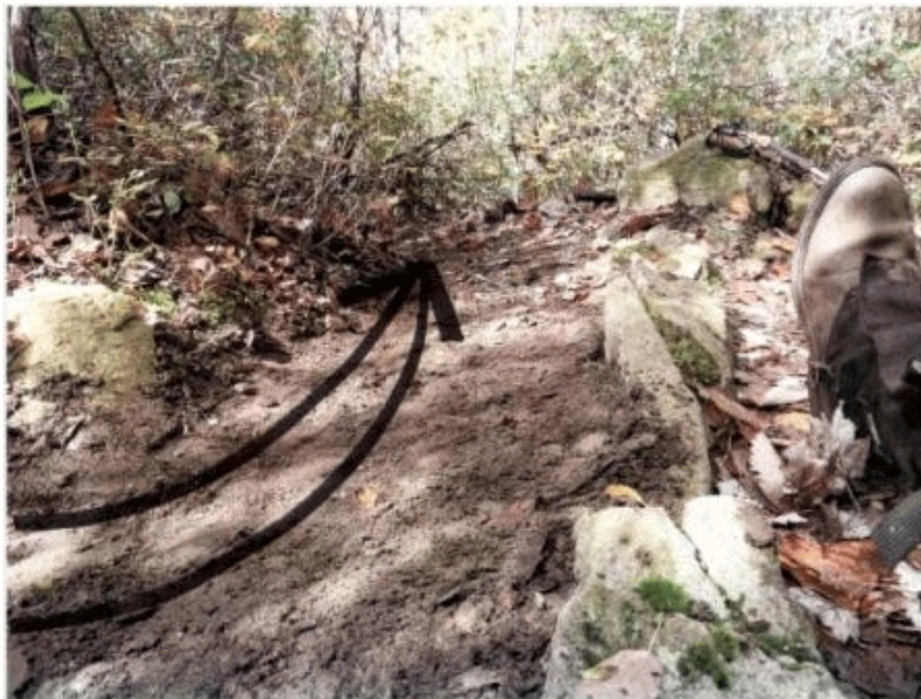
Water Flow Around the Grand Prix Curve into the Drainage Channel. Do not remove the dirt against the waterbar - it forms the Grand Prix Curve. Firmly tamp any loose dirt with your boots or the back of the grub hoe blade on a Pulaski, pick mattock, or cutter mattock.
