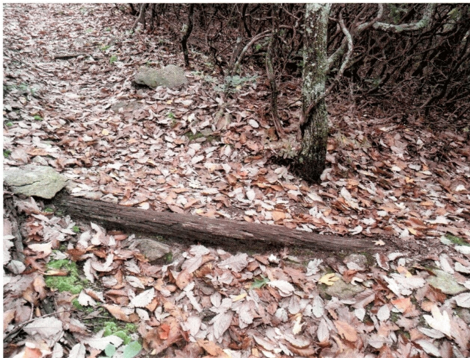
A Simple Water Bar before Maintenance
